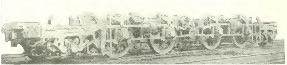
Articulated Truck of Electric Locomotive.
